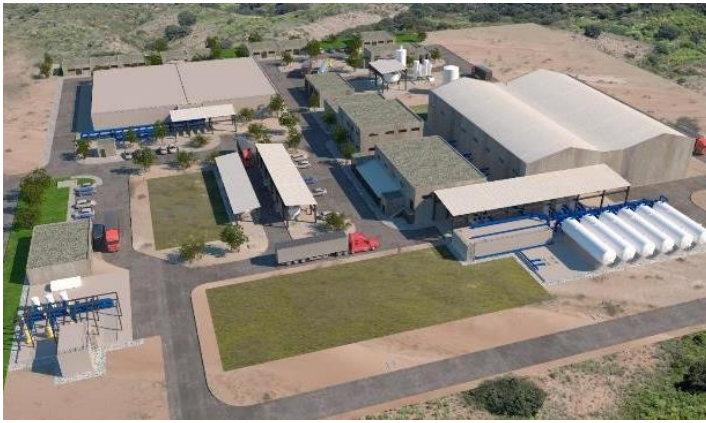
Future seawater desalination plant in Jaffna, Sri Lanka / Credits: SUEZ
