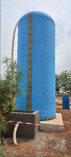
15 m treated water storage tank 3
