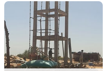
Construction works at Jidrel Mohguen
