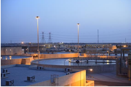
Wastewater treatment plant in West Doha, Qatar
