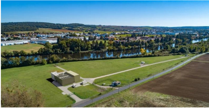
Boisseaux plant photo mock-up
