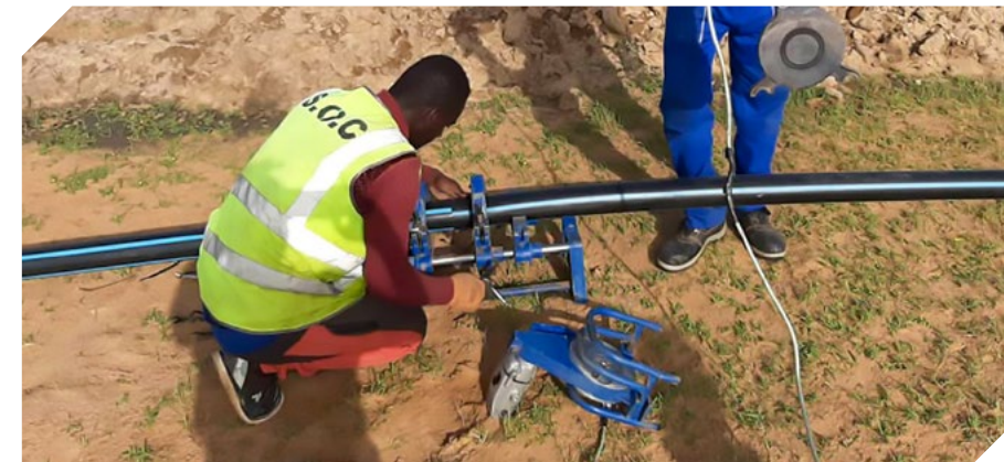
Technical service training is essential for the continuity of structures
