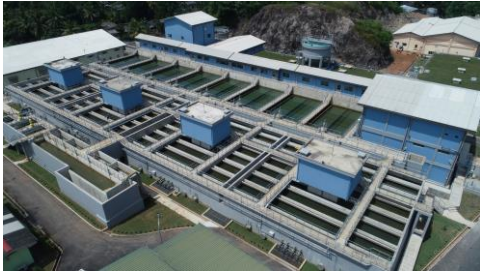
Kelani River Bank (KRB2) Water Treatment Plant in Colombo (Sri Lanka)
