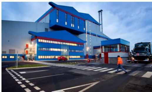
SUEZ's energy-from-waste plant located at Haverton Hill, Teesside
