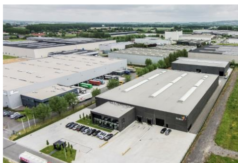
TIVACO's Plastic recycling plant
