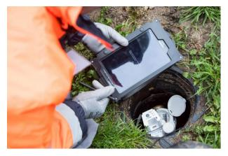
Installation of a smart water meter - © SUEZ
