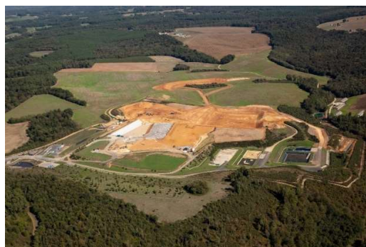
Aerial View of the Madaillan landfill – Copyright ©SUEZ
