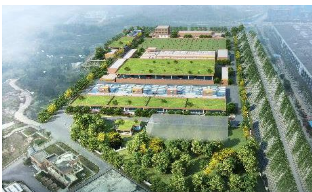
3D aerial view of Chongqing Yuelai WTP Phase IV project
