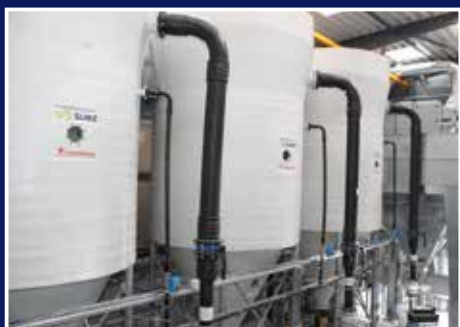
Marselisborg WWTP, Denmark capacity: 200,000 PE 2018
