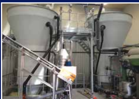
Herning WWTP*, Denmark capacity: 150,000 PE 2015
