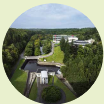
Eupen plant - la Vesdre, Belgium 2 700 m 3 /h
