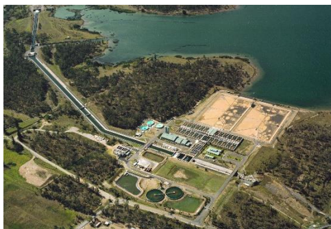
The Prospect Water Filtration Plant (PWFP)
